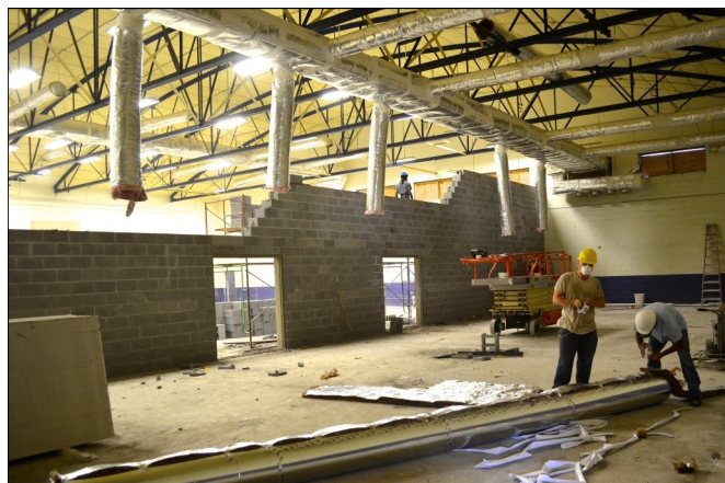
Renovation work is progressing quickly at the Howard Center. The photo above shows a wall being built in the gym area.
