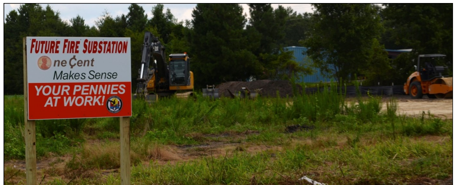
Fire substation sites are being prepared in Williams Hill and Yauhannah. A third is being permitted in Carvers Bay. These substations should be complete by mid-December.
