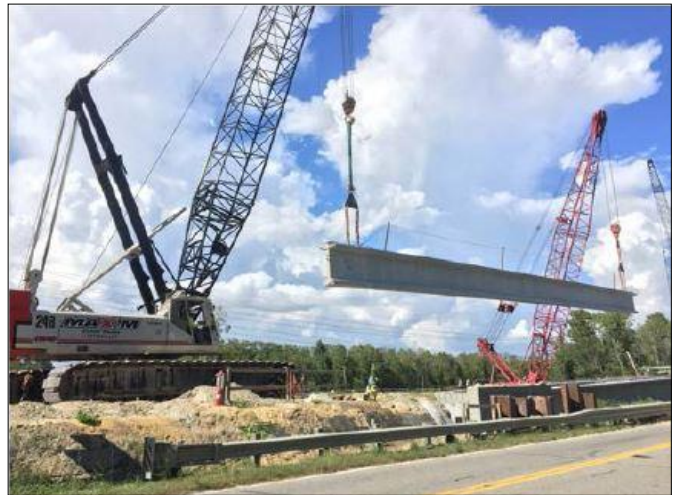
One of five girders is placed for the last span of the Yauhannah Lake Bridge. This span was not in place when the aerial photo above was taken.
