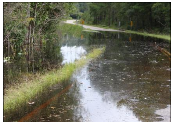
Flooding is shown on Sandy Island Road.
