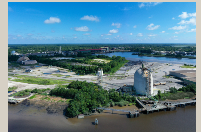
County lays out timeline for moving forward in Port Redevelopment Master Plan Process
