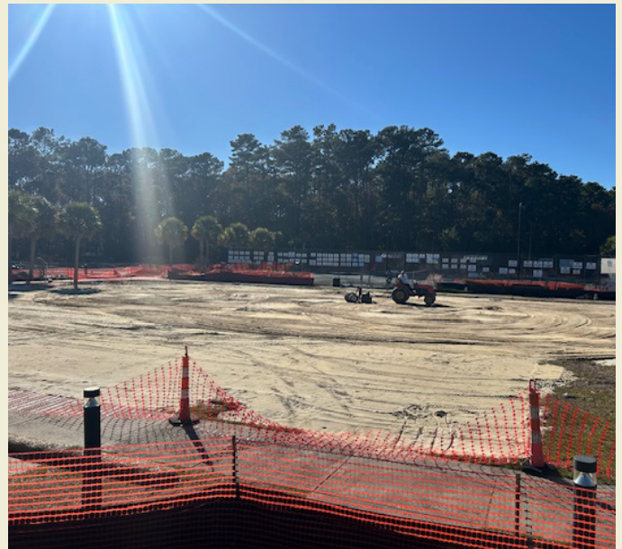
Construction of new tennis courts as seen from the center’s porch.
