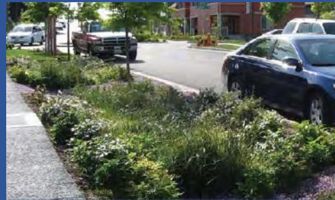
Example of using native vegetation to reduce runoff and improve water quality (Source: United States Environmental Protection Agency)
