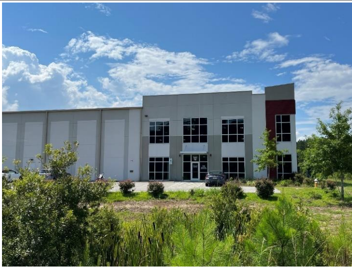
Industrial building, Georgetown County Business Center
